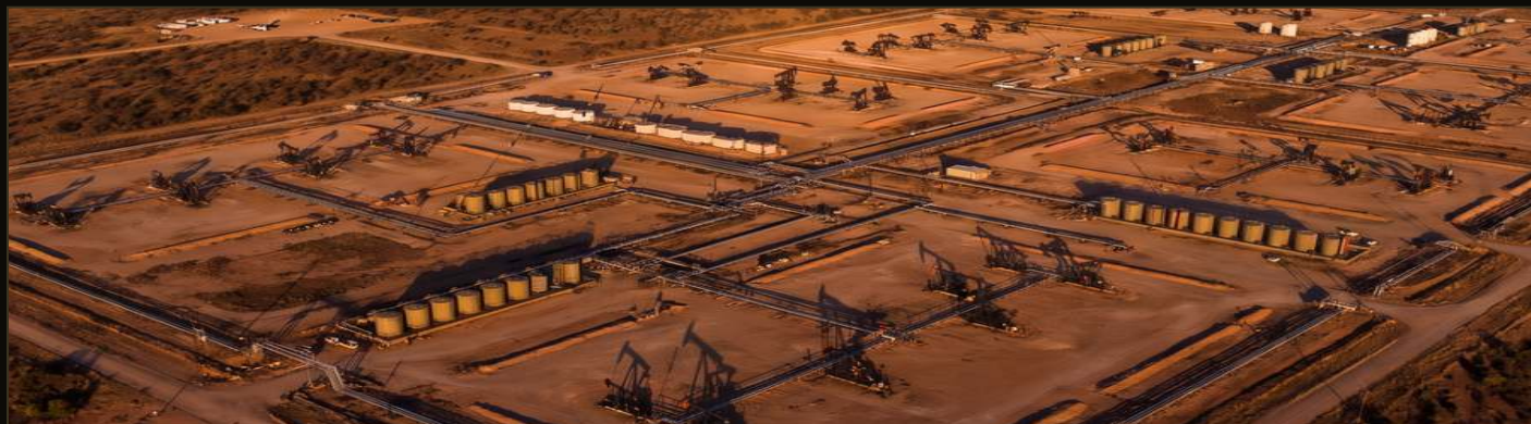
Aerial view of producing wellsite infrastructure, Loving County
