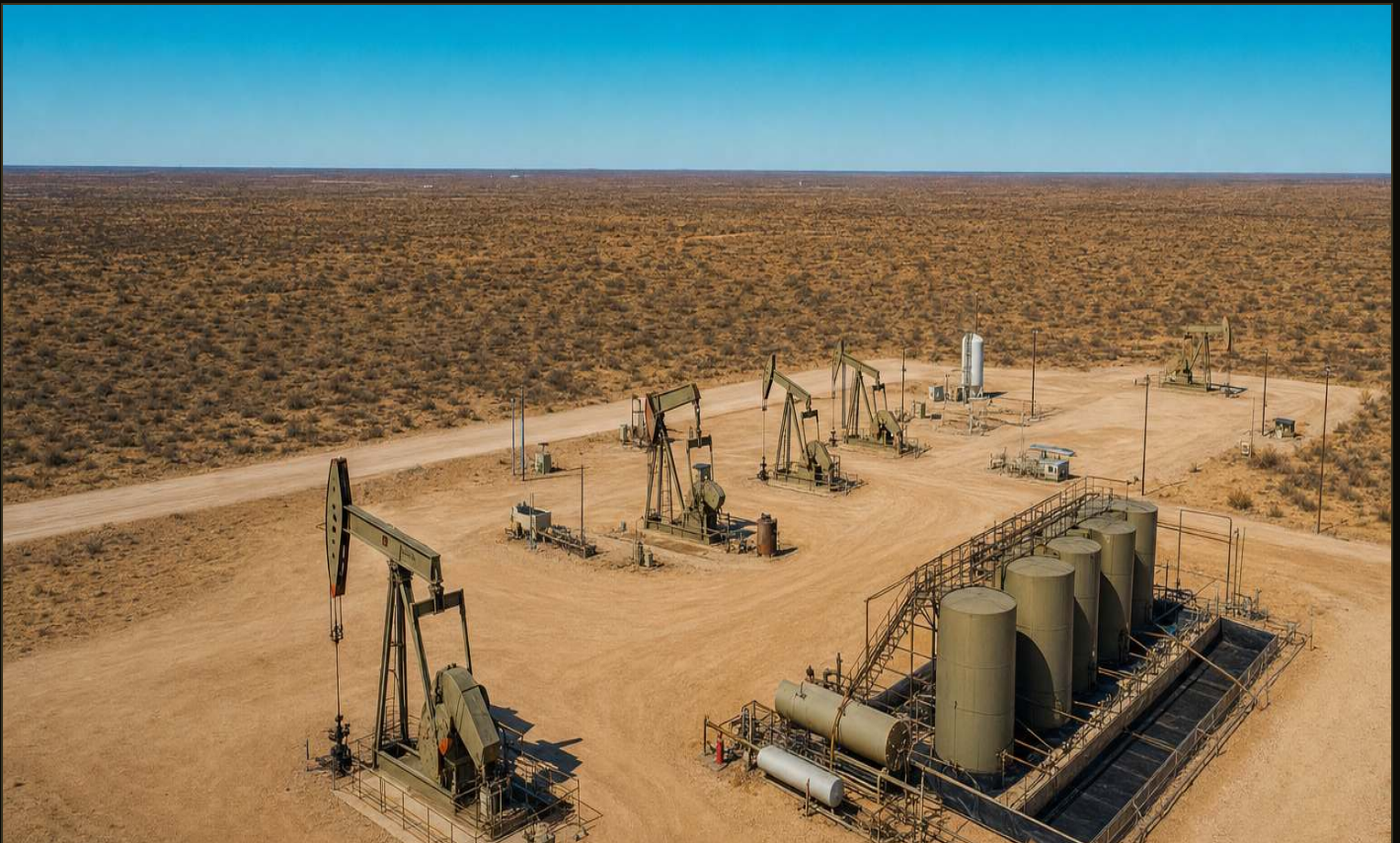
Multi-well pad site, Midland Basin
